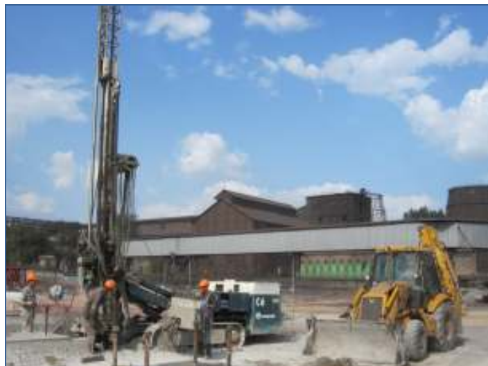
Figure 2 – Execution of test jet columns by Casagrande C6
