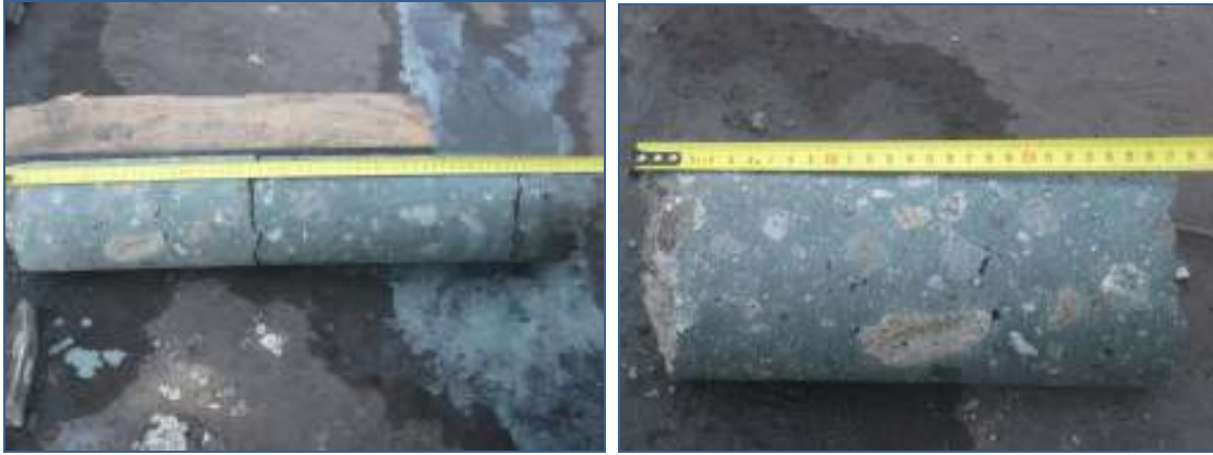
Figure 4 – Core from JC-1 column (total length of core parts - 640 mm)
