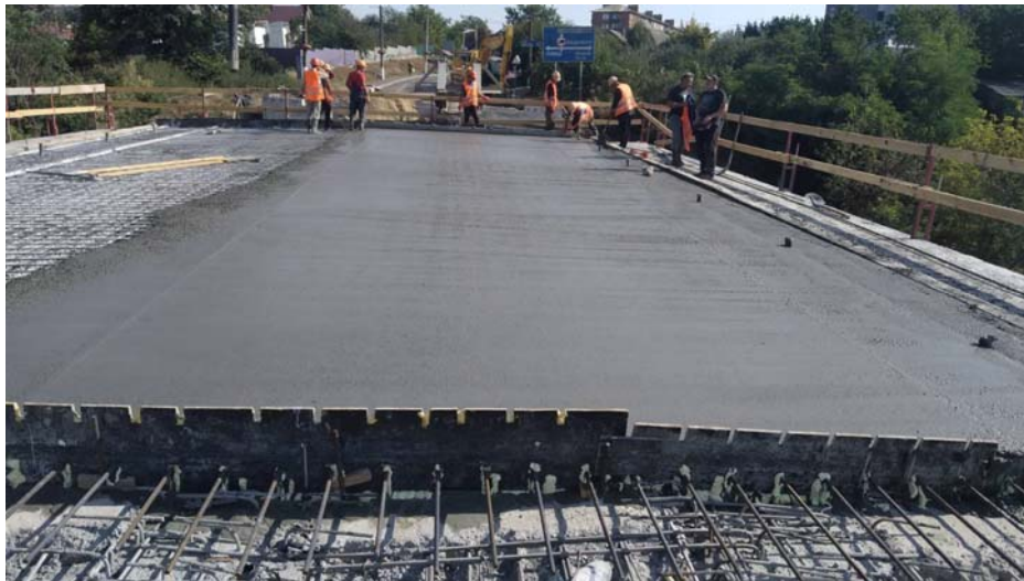
Figure 2 – Concreting of the overhead slab of the girder structure using SCC based on superplasticizer
