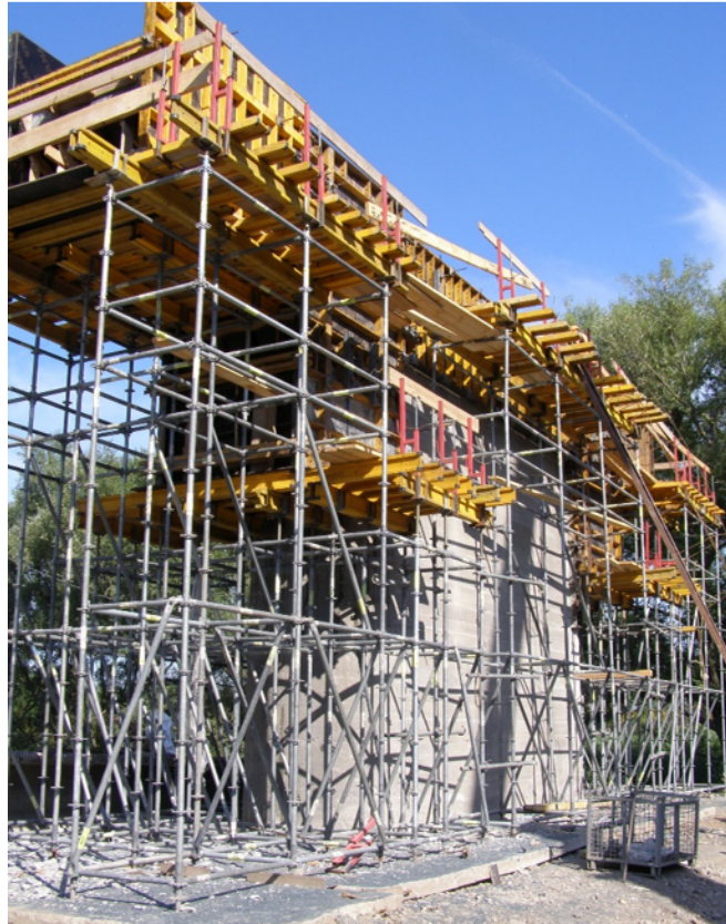
Figure 1 – Example of a high-rise formwork system for the reconstruction of a bridge supports. Concreting works were carried out using SCC
