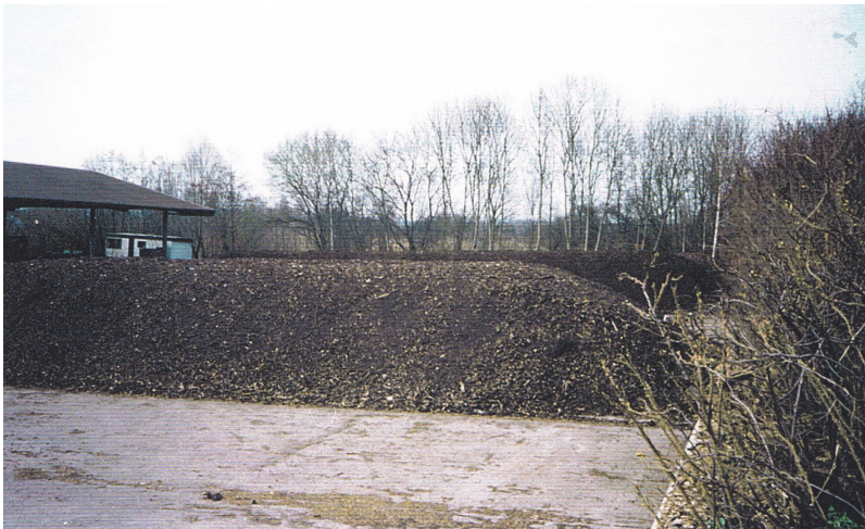
Figure 6.14. Aerobic composting plant
