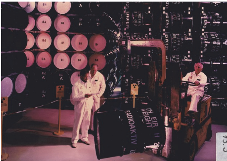
Figure 6.16. Storage room for medium and low level radioactive waste.
