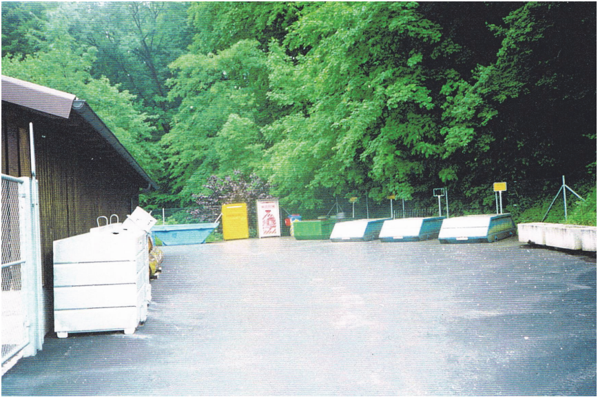
Figure 6.6. Modern collecting center for separate collection of paper, waste oil, cardboard, inert material, glass, metals, construction waste, hazardous waste, electronics.
