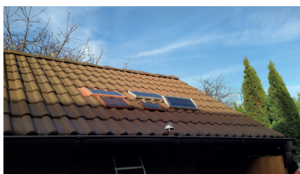
Fig. 7. Shading of the front two panels by the roof of a family house
