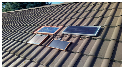
Fig. 2. Detail of the model installation
