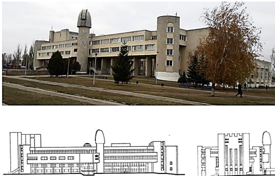
Fig. 8. General view of a full-scale object № 2
