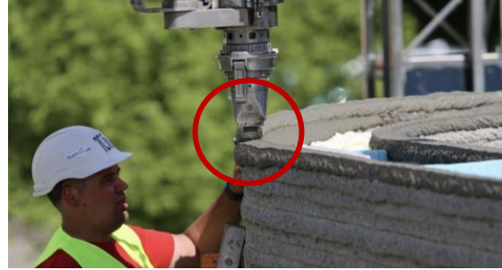
Fig. 2. 3D printer nozzle
