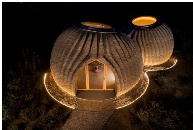
Fig. 3. House built using clay and 3D printing
