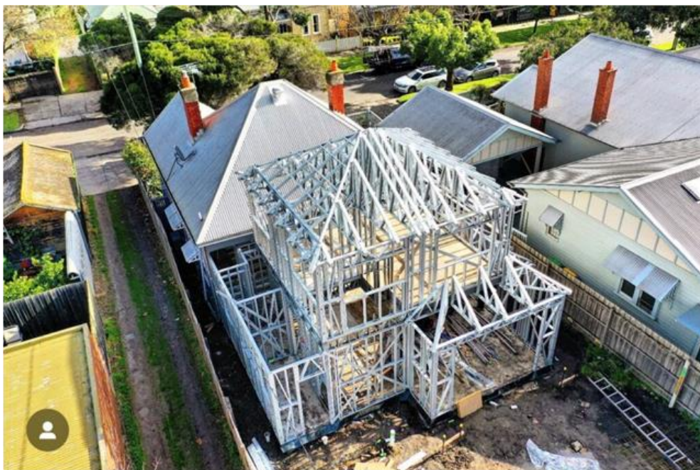
Picture 1. The example of usage LGSF in civil construction
